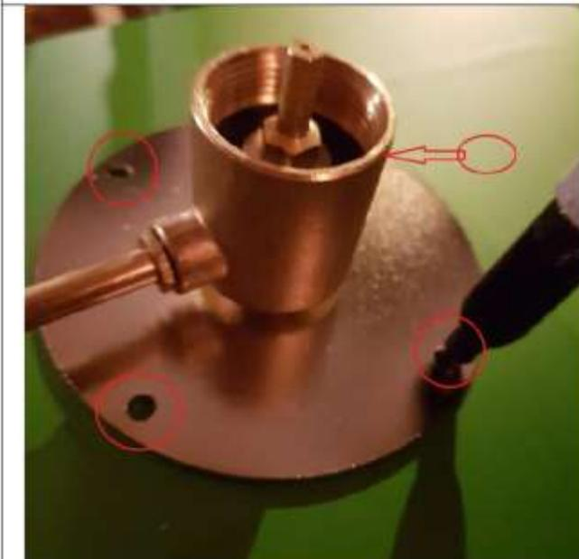
3) Mark 4 holes with pen and drill out with a small drill bit that is smaller than the screws.
